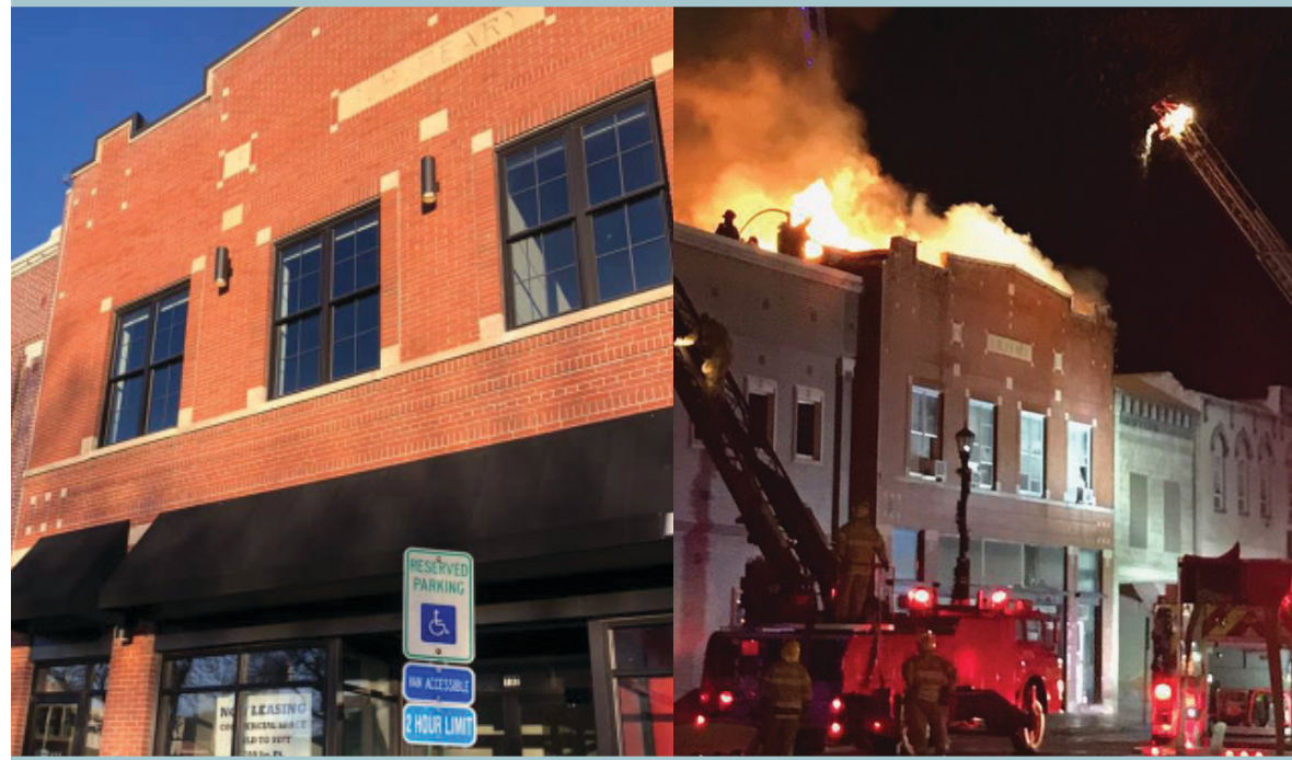
(Above) The IH Feary Building (132 S. 5th St.) suffered a substantial fire but has now been rebuilt into seven executive apartments and soon to be Jimmy John's restaurant.
