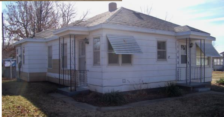
Before and after photos of home rehabilitated in Falls City, Nebraska.
