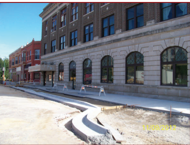
Falls City DTR improvements
